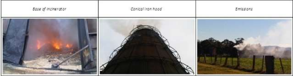
Image 4. Conical incinerator at MecTech Hardwood Sawmill
