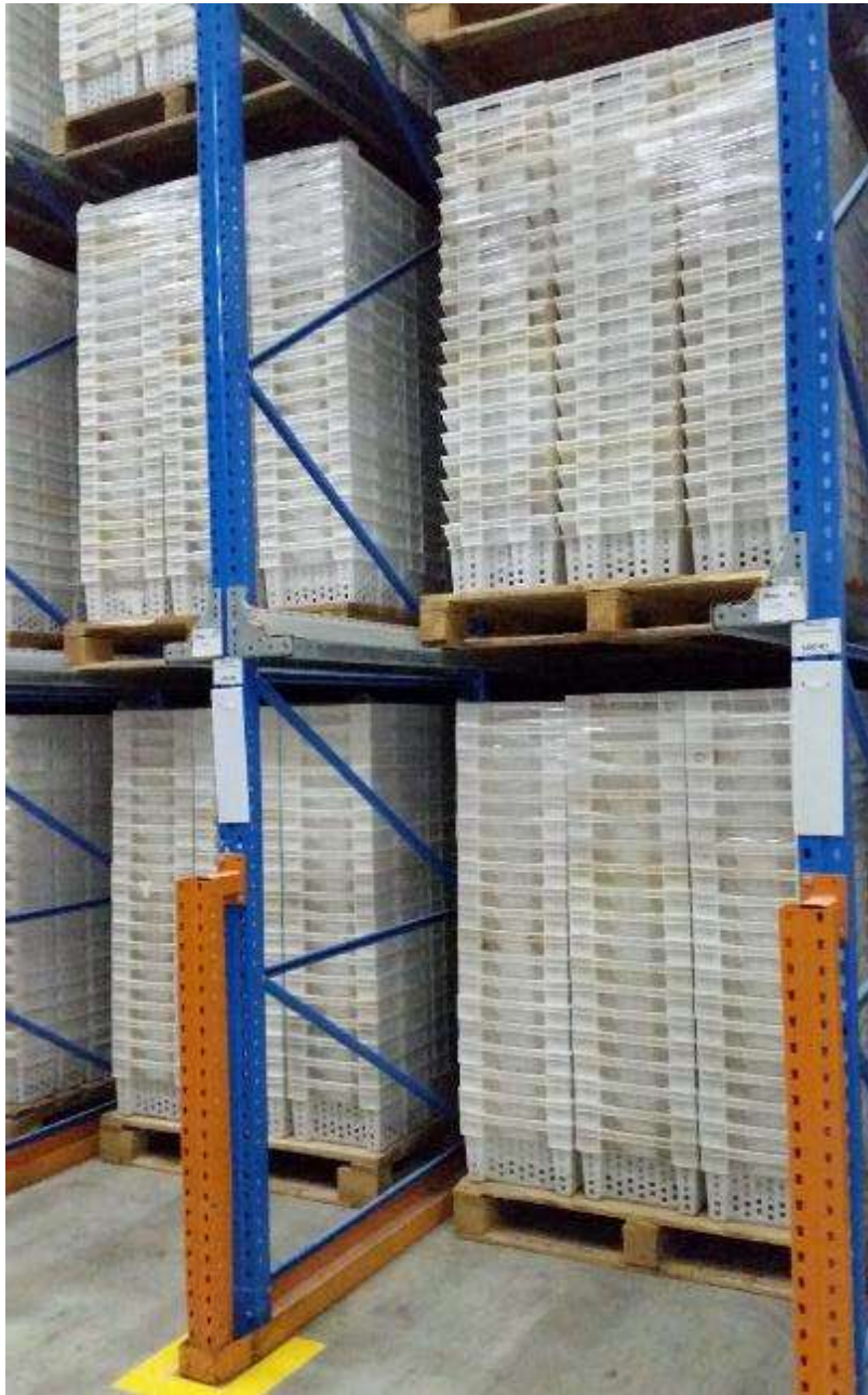
Figure 18 Cold room for storage of dates
