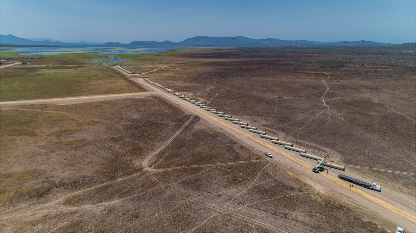
Image: Stage 1 and 2 of Burdekin Haughton Pipeline. Source: Infrastructure Australia, n.d.
