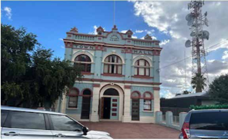
LEFT: Restored Nyngan Town Hall
