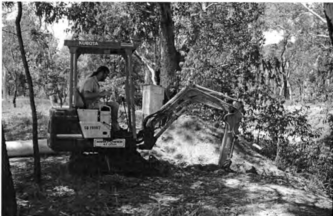
Figure 2 Digging the trench at Swift Creek with the Mini Excavator
