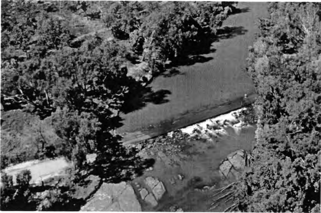
Plate 24: Cahills Crossing, East Alligator River during the dry season. Note that the crossing has been built on a foundation of bedrock and acts as a weir during the lower part of the tidal cycle. Slide No. 21 Mike Saynor, 2/6/97.
