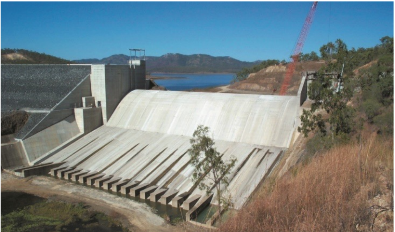
Image: Awoonga Dam. Source: Sunwater.
