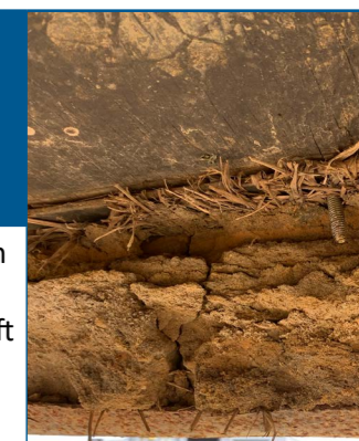
soil under container
