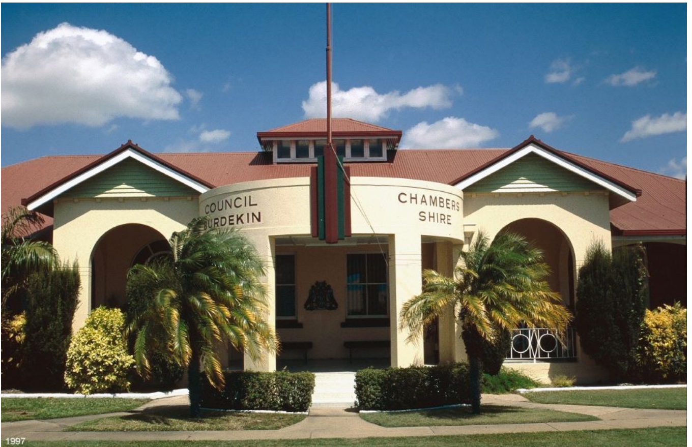
Image: Burdekin Shire Council Chambers. Source: Burdekin Shire Council.
