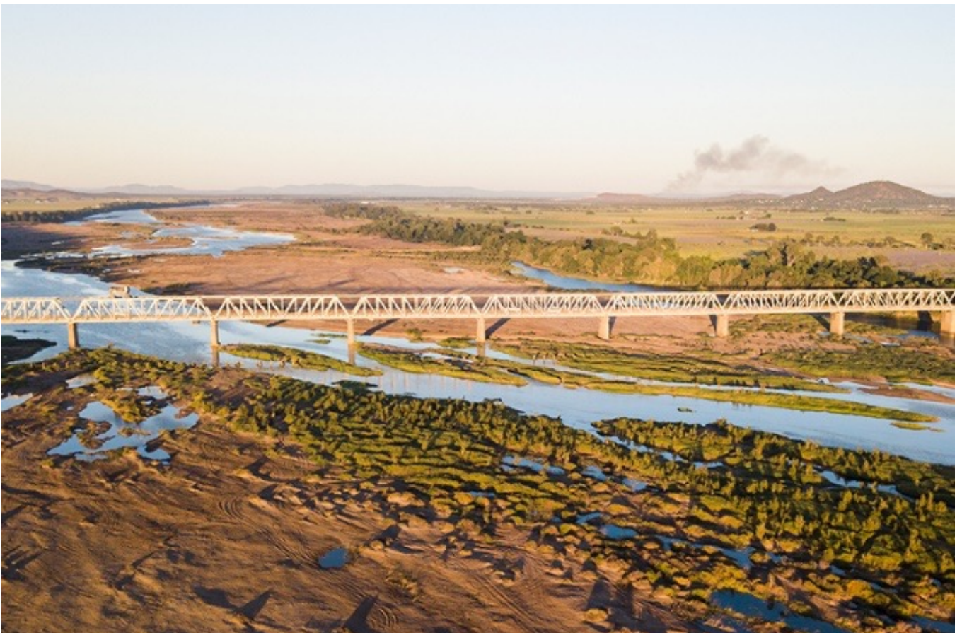
Image: Sunset over the Burdekin Bridge. Source: Burdekin Shire Council.
