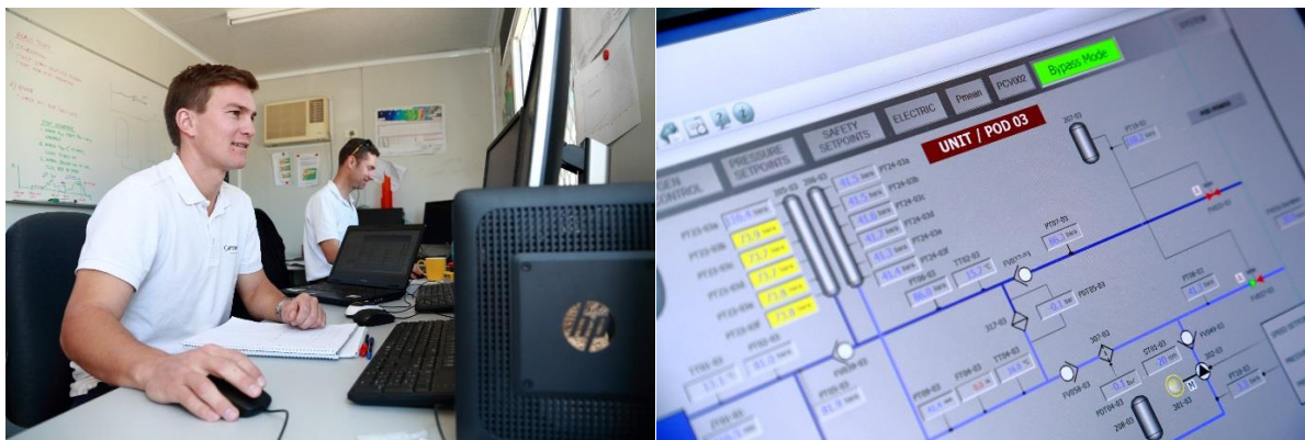
Plant Operators and Operator's Plant Control Interface
