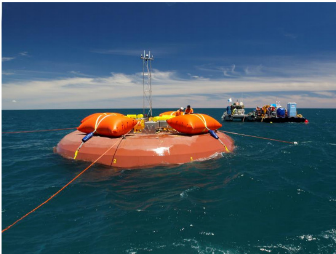
CETO 5 unit during installation at the Perth Project site
