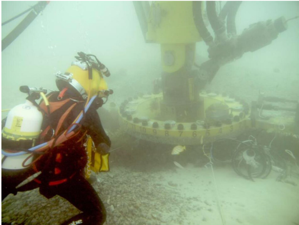
Installation of the CETO 5 unit into the offshore foundation
