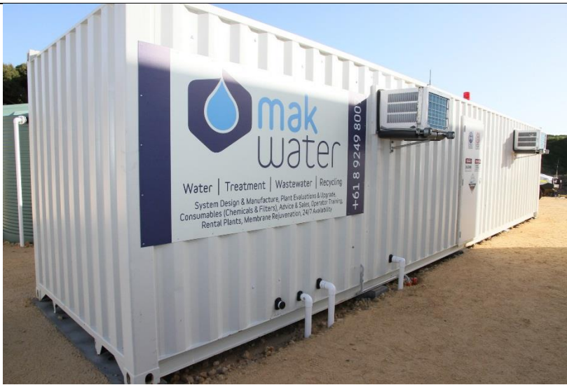
Containerised Desalination Plant
