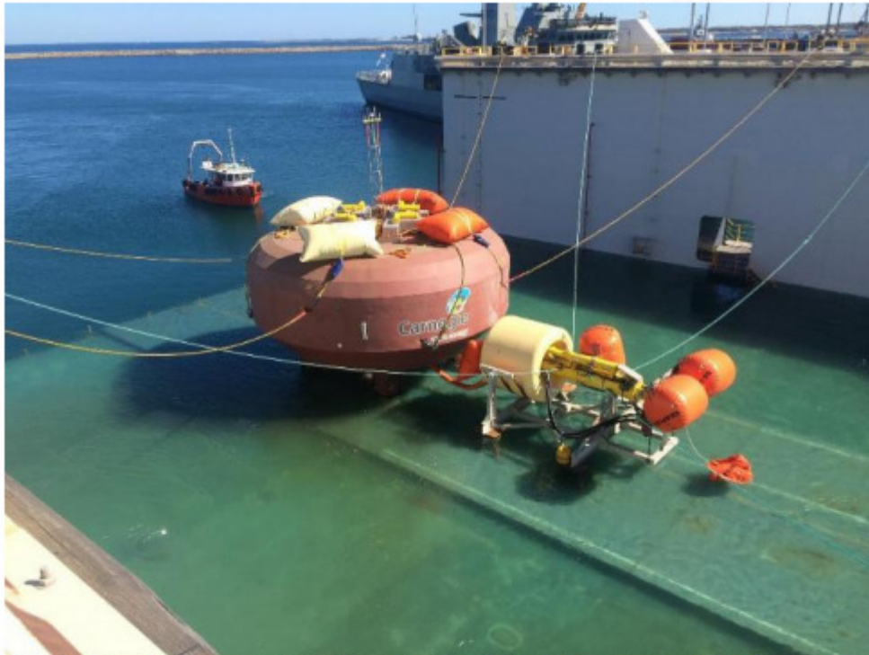
CETO 5 Unit #3 being lowered into the water on the floating dock at the Australian Marine Complex, Henderson, WA
