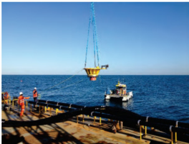
Installation of a Foundation Connector (left) and in place on an offshore foundation (right)
