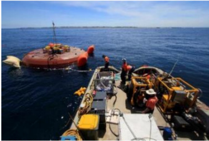
The second CETO 5 unit being installed off Garden Island, Western Australia
