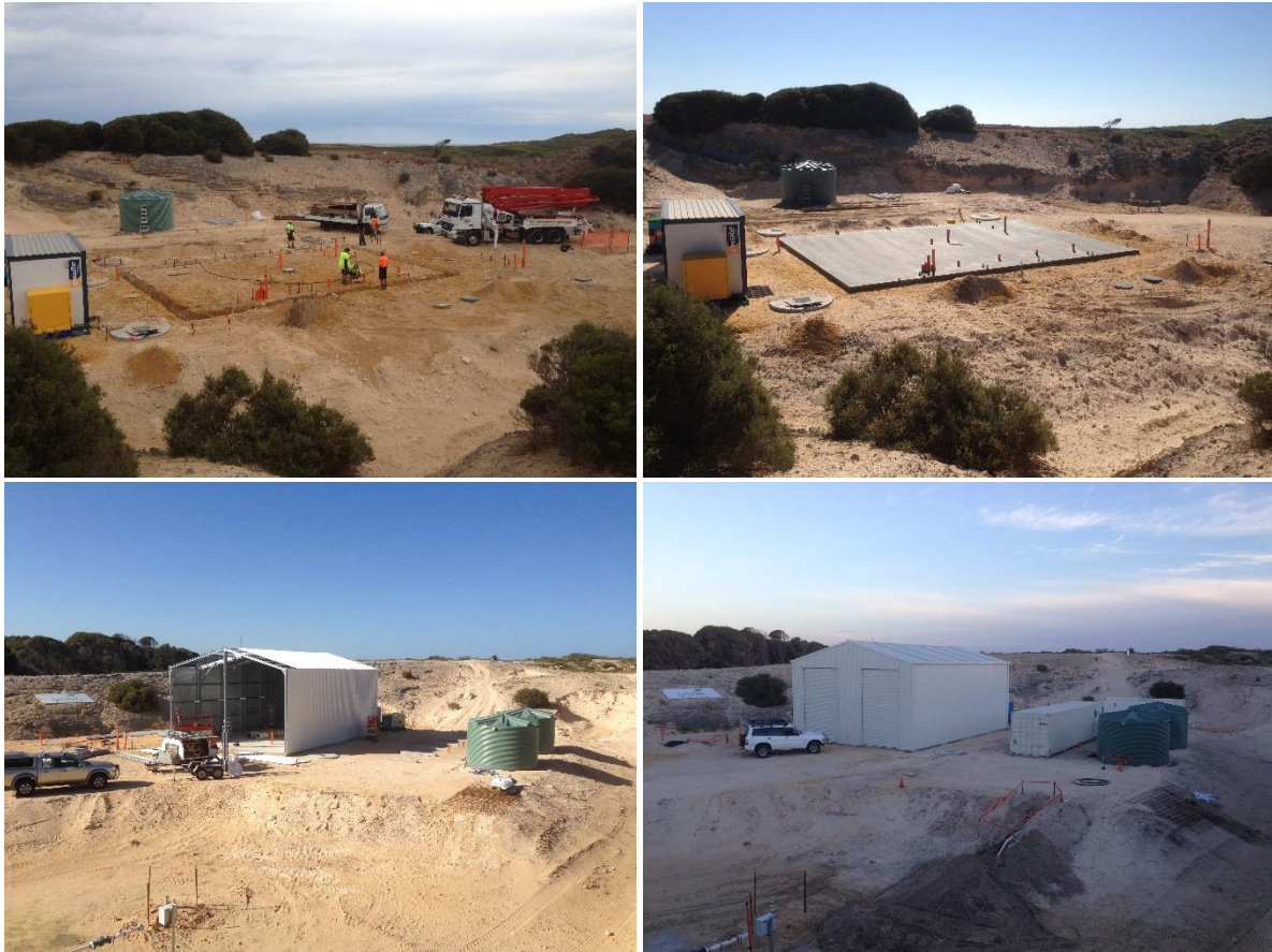
Construction of Onshore Plant Building
