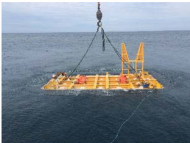
Offshore installation of Pod #2 mudmats and lower foundation connector #2
