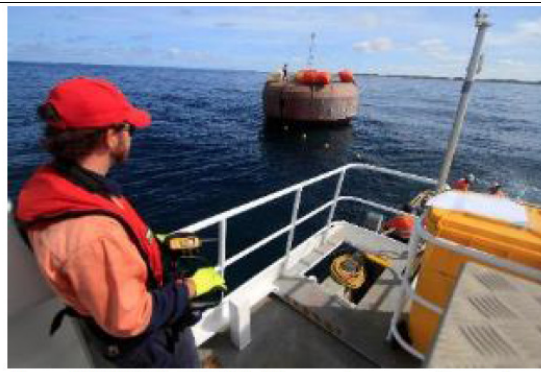
CETO Unit 2 prepared for deployment quayside along CETO Unit 3 (L), Carnegie operations team member controlling position of Buoyant Actuator from deployment barge (R)
