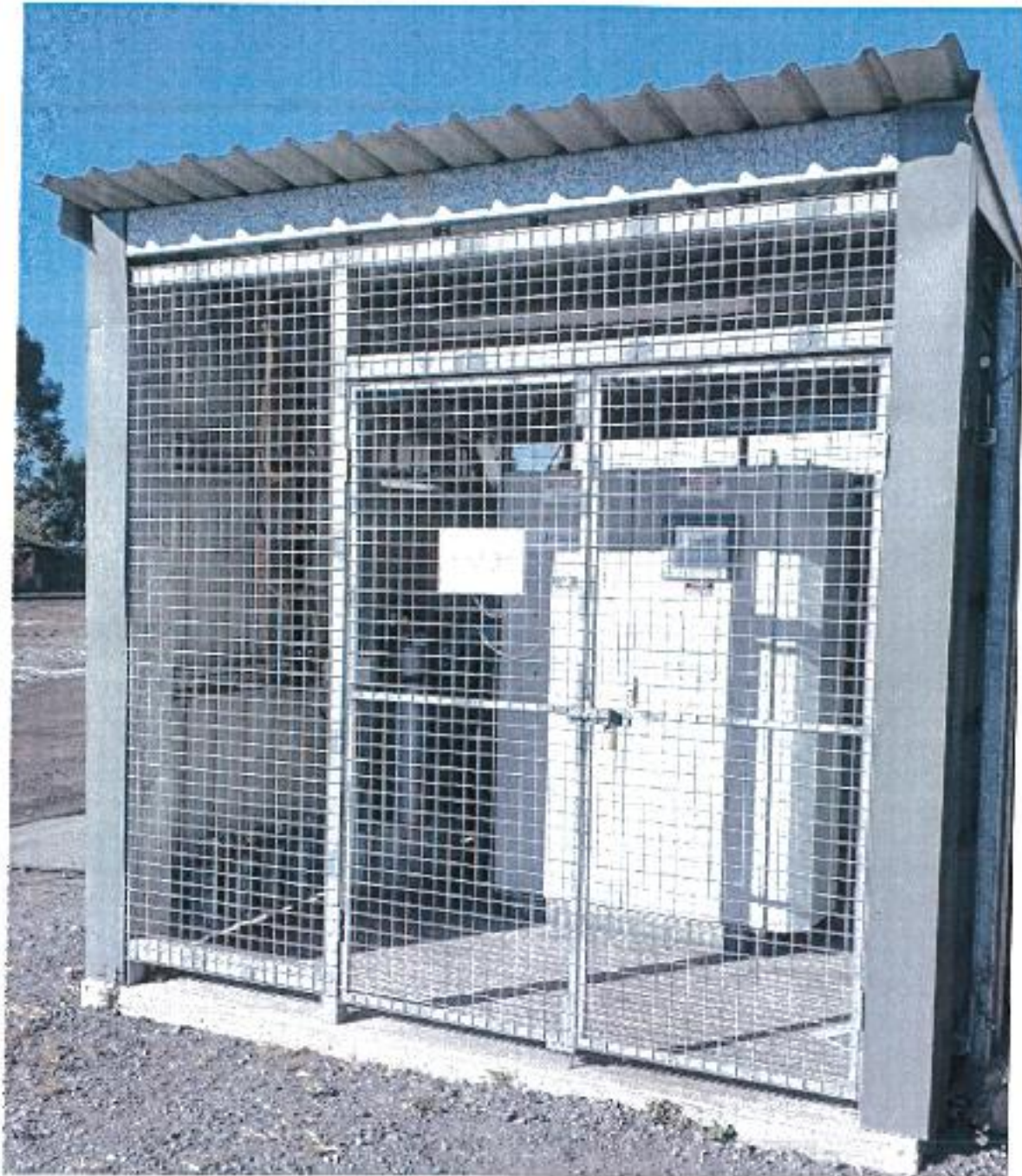
Figure 4 - Tube Bundle enclosure
