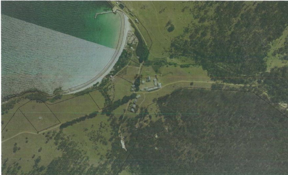
Figure ii: 2007 CMP plan of listed place. The boundary appears to relate to a contour line. The indication of buildings is nominal and does not reflect the site layout.
