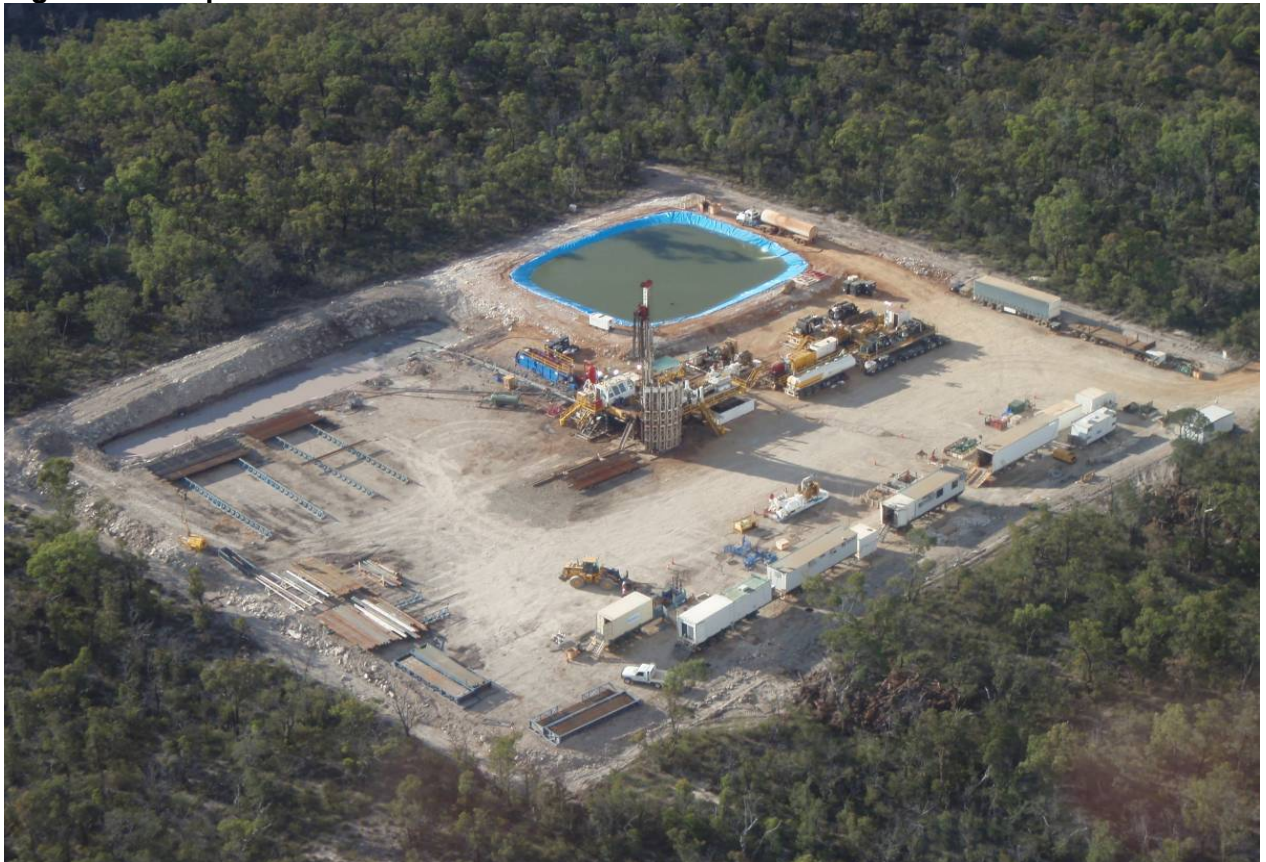
Figure 3: Multiple well site under construction
