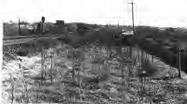
Photo 7. General view of Transmission line route along railway line between Raglan and Bathurst. Looking west towards Railway Bridge.
