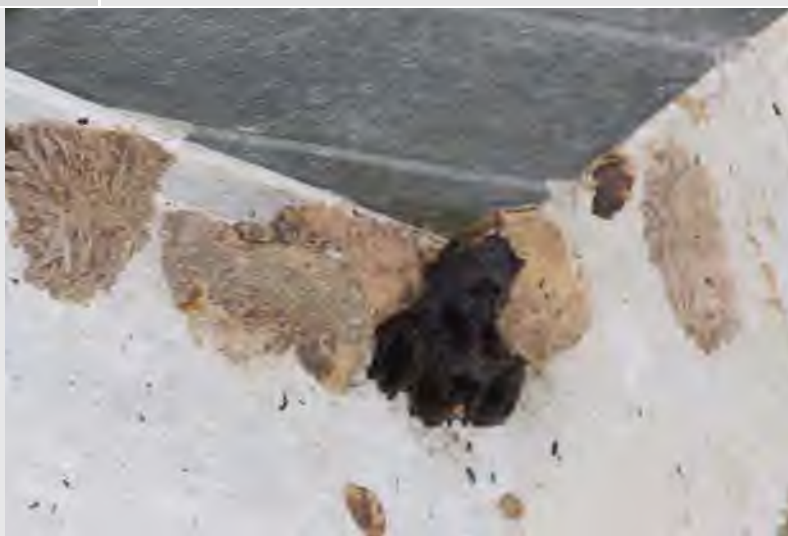
Roosting bats and swallow nests under Badgerys Creek Road bridge.
