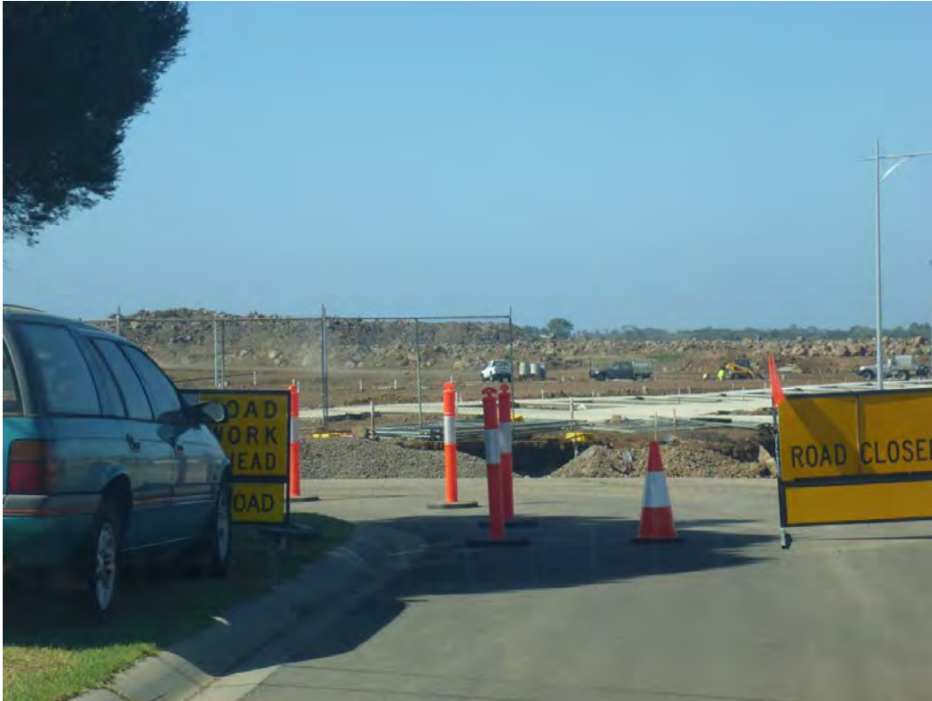
Blackforest Road, Wyndham Vale, current rock stockpiling
