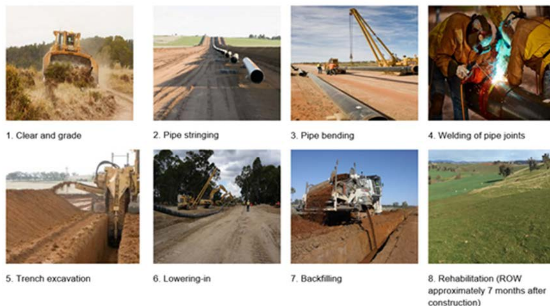
Figure 5 Pipeline construction sequence
