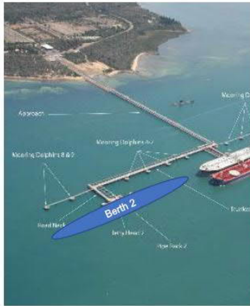
Figure 2 View of Crib Point jetty from south east
