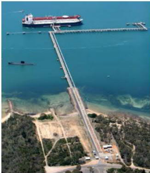
Figure 1 View of Crib Point Jetty
