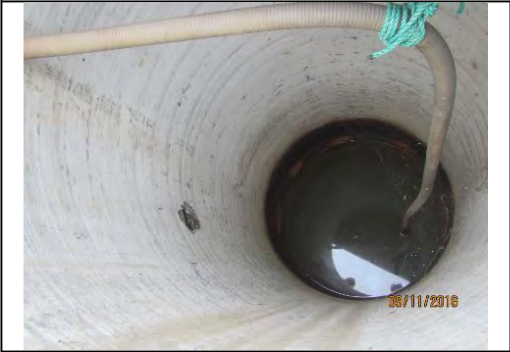
Photo 18: View down a concrete lined groundwater bore (located adjacent to airport)
