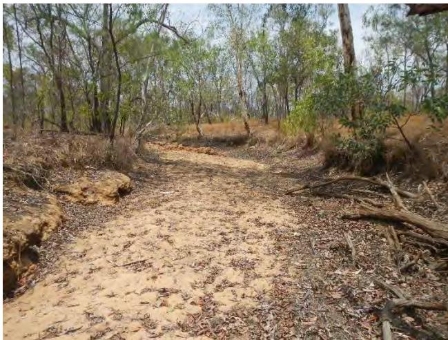
Figure 15 Bank erosion along Jones Creek, which could be accelerated from increased water runoff and sand accumulation in the bed that promotes channel widening and bank erosion.
