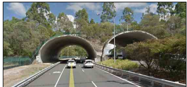
Photo 1. Google Earth photo of Compton Road overpass.
