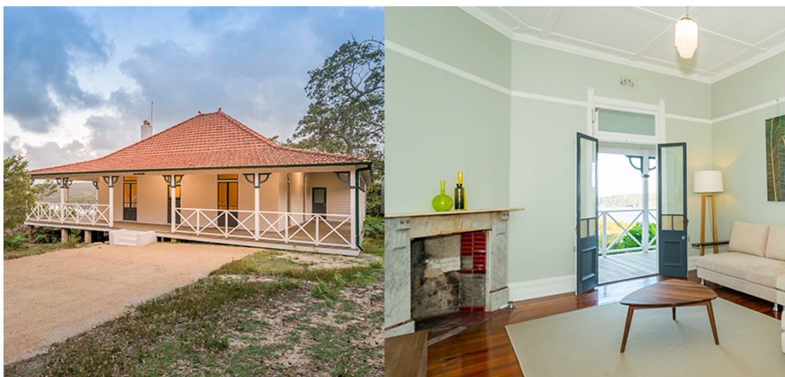
Figure 5.6: Examples of Eco cabins at Tidal River Wilsons Promontory Victoria (source: Parks Victoria) and boutique accommodation at Hilltop Cottage, Royal National Park NSW (source: NSW National Parks and Wildlife Service)
