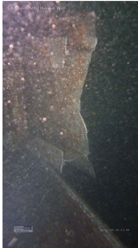
Photo 3: This photo shows the buckled starboard hanger side plating forward to the parted structure.
