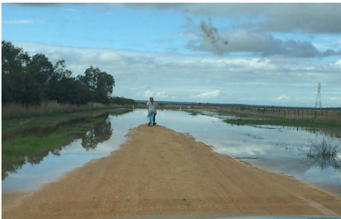
Figure 3 Flooding at Harriott Road 7
