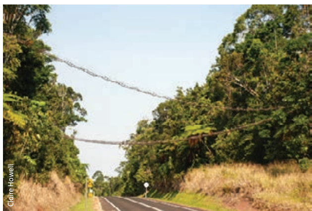
Possum bridge, to allow animals to move between forest fragments and maintain connectivity of populations.
