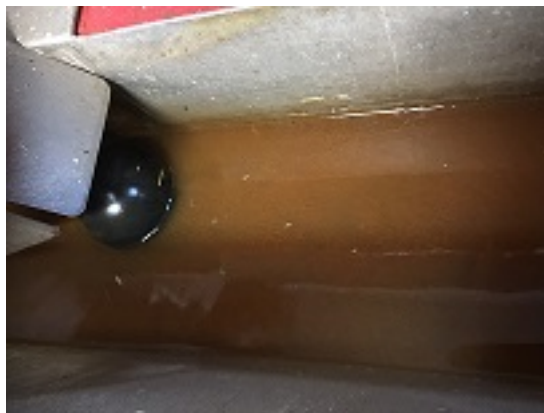
Figure 6. Fouled water trough
