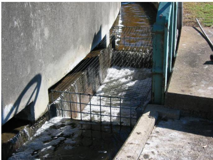
**Fig. 1.** Shallow channel surrounding secondary treatment tank at Wynnum waste water treatment plant, showing wire mesh in place over sump draining to tertiary tank.
